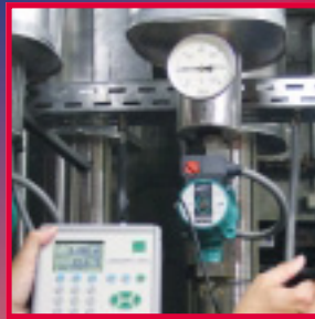
Testing a heating plant
