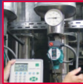
Testing a heating plant
